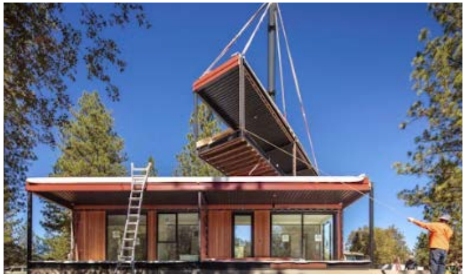
New housing module lifted into place by crane on a Connect Homes market-rate house
