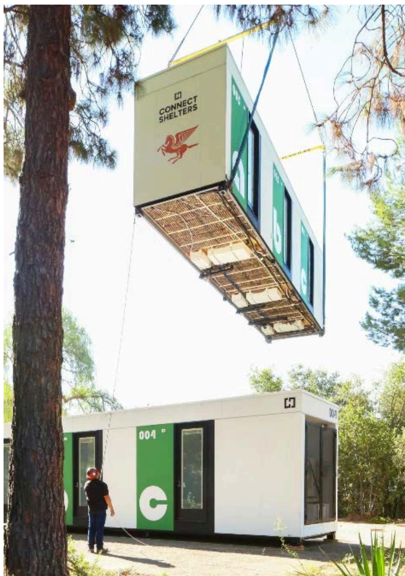
Connect Shelter unit lifted by crane
