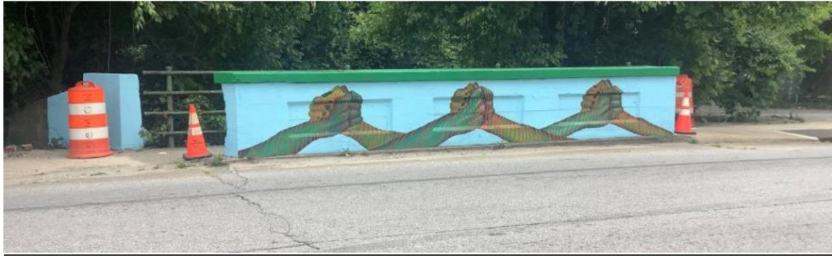
Murals Over Joseph E. Boone Bridge
