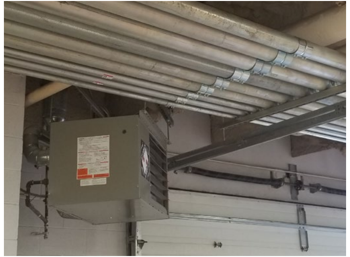
Overhead Elec Conduit Installation at Moxey Rigby
