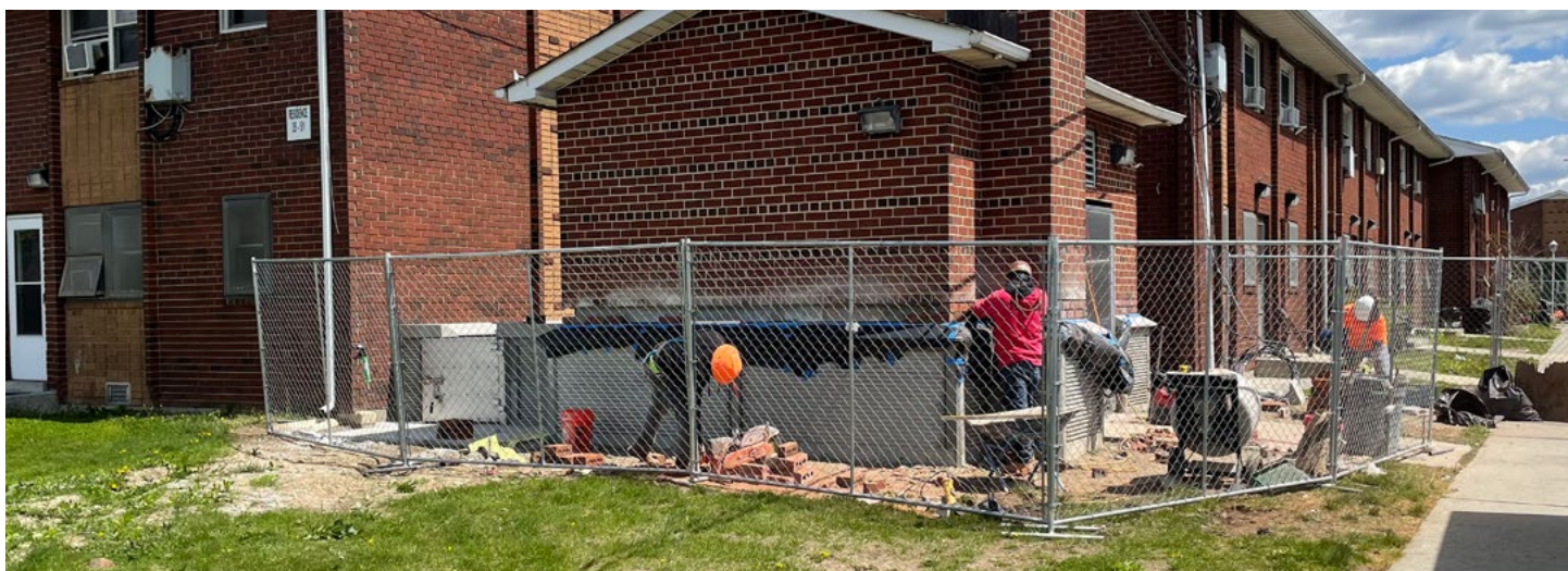
Construction at Inwood Gardens
