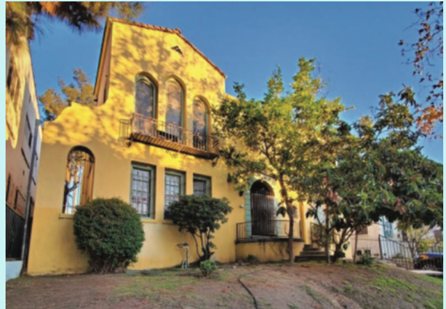
Beverly Vermont CLT and Brilliant Corners collaboration project in LA
