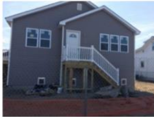
159 Radcliffe Road, Island Park – before and after
